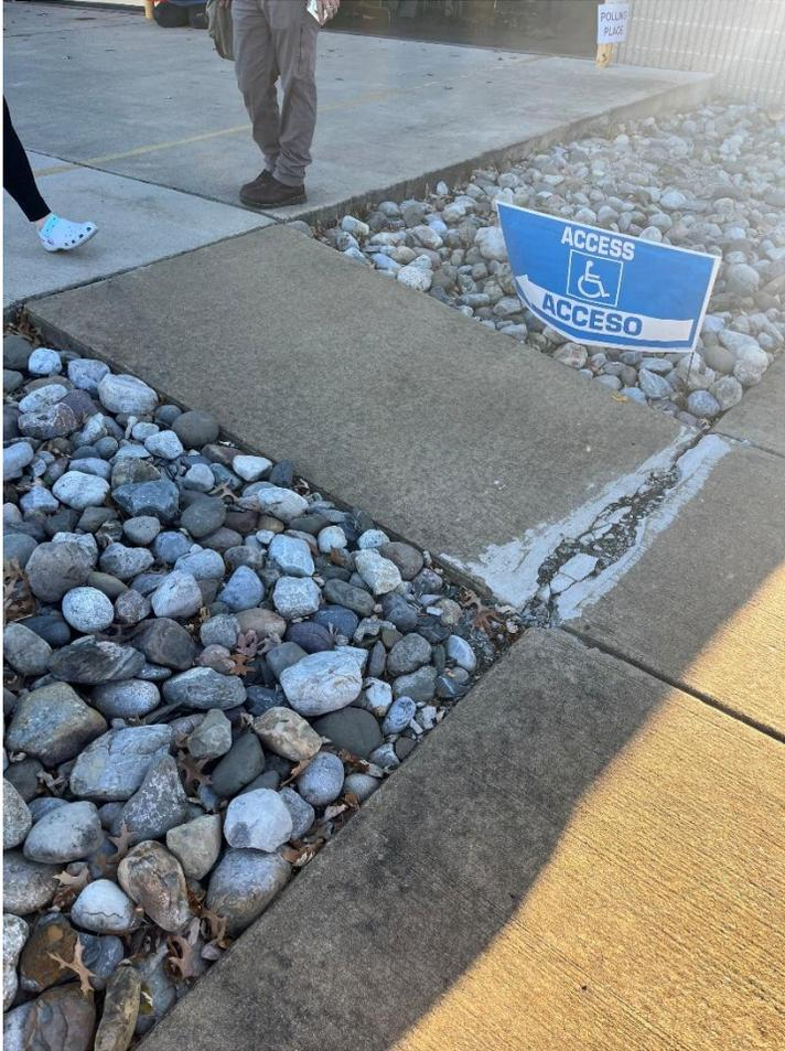
Poll monitor at **Aetna Fire Station in New Castle County** noted a large crack in the sidewalk ½ inch in width as well as a large crack at the base of the accessible entrance’s ramp, which would make it difficult to pass for a wheelchair-user.
