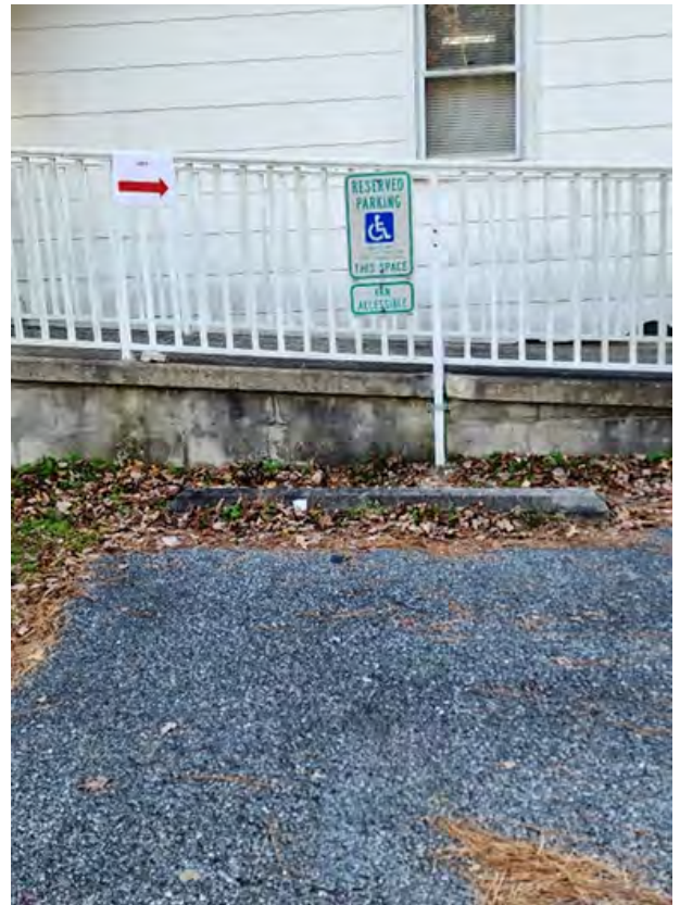
Loose, unstable gravel; no demarcation of spaces or aisle, sign too low. (Polling Place: Redden Community Hall)
