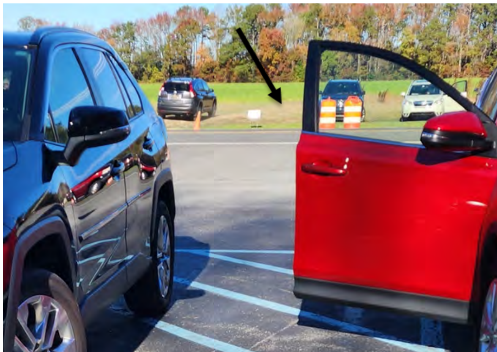
Insufficient parking: voters were instructed to park on the opposite side of the road and to walk across the busy highway to the polling place. The only spaces marked accessible were less than 96" wide and shared an access aisle. (Polling Place: Mid Sussex Rescue)
