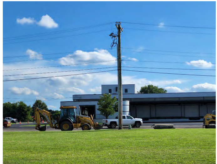
View from front (north); construction limited the survey
