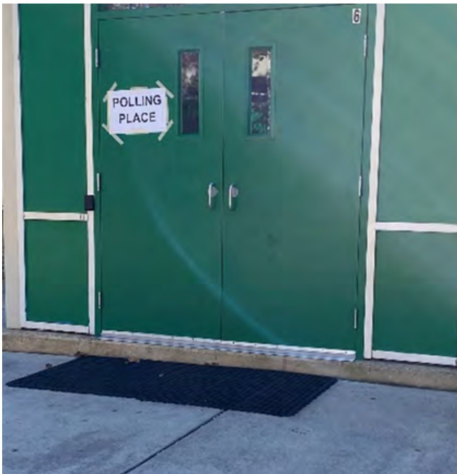
Threshold exceeds maximum height of \frac{3}{4} " (Polling Place: East Side Charter School)
