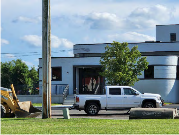
Stairs visible; ramp on left begins on eastern side
