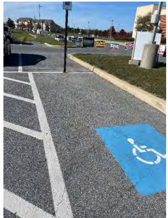
Space less than 96" wide. (Polling Place: Dover High School)
