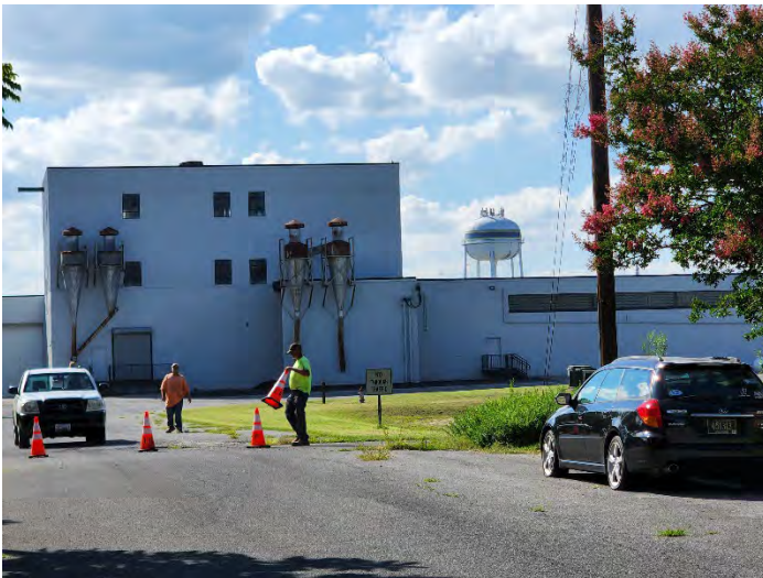
View from end of Allen St (east side of the building)
