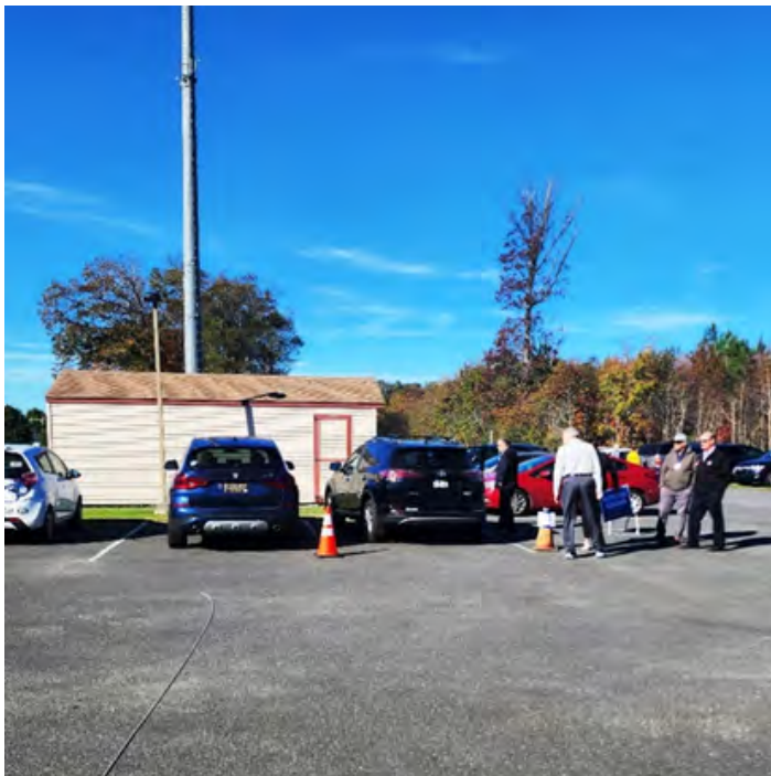
Cones with no sign, no access aisle. (Polling Place: Lewes Fire Hall)
