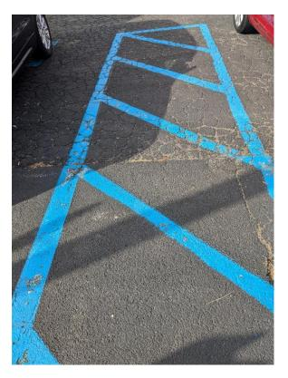
**Peniel United Methodist Church in New Castle County.** Spaces were ADA compliant for width, access aisles, signage, and proximity to entrance. However, parking surface was cracked and uneven.
