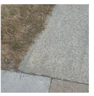
**P.S. DuPont Middle School in New Castle County.** Poll monitor indicated that curb cut from pavement to the sidewalk was uneven, with changes in elevation of 1-2 inches.
