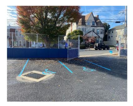
**Pulaski Early Education Center in New Castle County.** None of the marked accessible spaces at this site were compliant for width or access aisle. A grate and an open fence door protruding into one of the spaces could cause obstacles.
