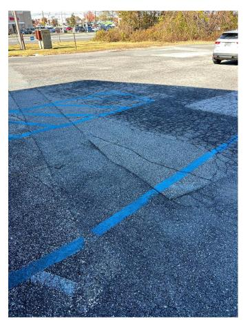
**Eden Support Services in New Castle County**. Poll monitor noted many cracks and uneven surfaces in the marked accessible parking area and route.
